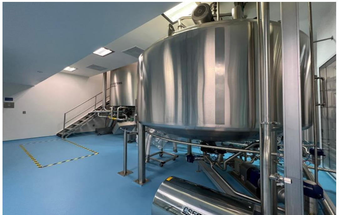
Semi-solids Manufacturing Line
