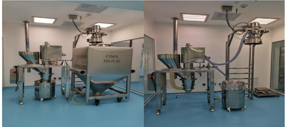
Sifter and Vacuum System ( Solids Manufacturing Line )
